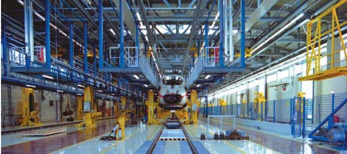
Thirty-nine radiant panel modules were installed, with a length of 1,147 m. Placement of the panels required a large amount of skill in order not to be in the way of the crane rails running the entire length of the hall over the three sets of tracks.
