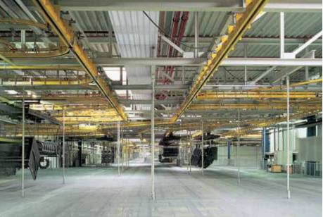
A total of 419 Zehnder radiant ceiling panel elements were installed in the new assembly halls. Their suspension was integrated without difficulty in the complex production lines of the fully automated paint shop.
