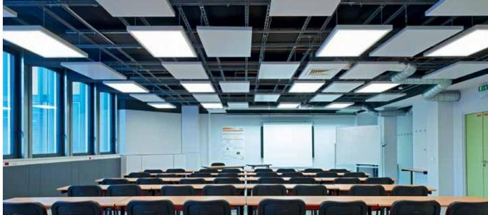
The building complex extends over a total area of 70,000 m<sup>2</sup>. 12,000 modules of the Zehnder radiant ceiling system were installed over 7,275 m<sup>2</sup>.
