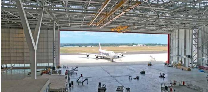
17,000 m² floor space and a ceiling height of up to 42 m: an enormous challenge for Zehnder radiant ceiling panels. The principle of thermal radiation takes full effect here, particularly considering that the heat is required mainly in the lower area of the hall.
