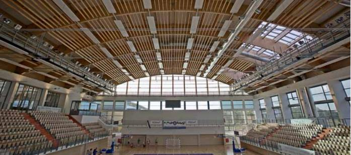
In order to heat the 5,000 m² large hall evenly and efficiently, the decision was made to choose Zehnder radiant ceiling panels. A total of 372 m² of perforated radiant panels for noise reduction were installed on the wooden structure which supports the roof of the hall.
