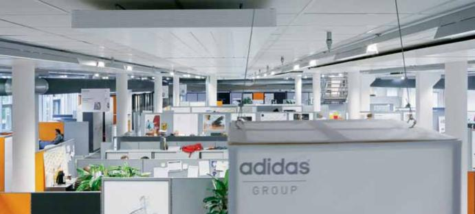
Areas where warm air collects in larger quantities must receive more cooling – and vice-versa. Thanks to the high radiation component of the flat panels, a comfortable indoor climate is achieved with high efficiency.
