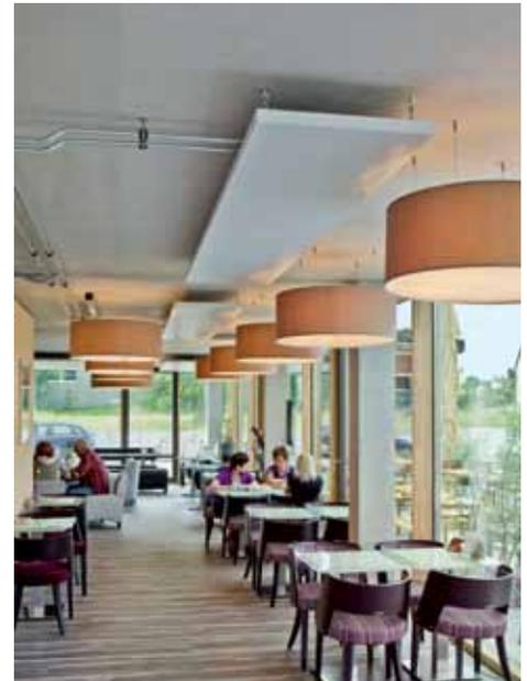
The climate in all of the office areas, including the cafeteria, is controlled with Zehnder radiant ceiling panels. The lightweight panels with natural graphite ensure particularly rapid, even and efficient temperature distribution.
