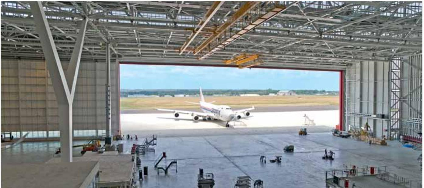
17,000m<sup>2</sup> floor space and a ceiling height of up to 42 m: an enormous challenge for Zehnder radiant ceiling panels. The principle of thermal radiation takes full effect here, particularly considering that the heat is required mainly in the lower area of the hall.
