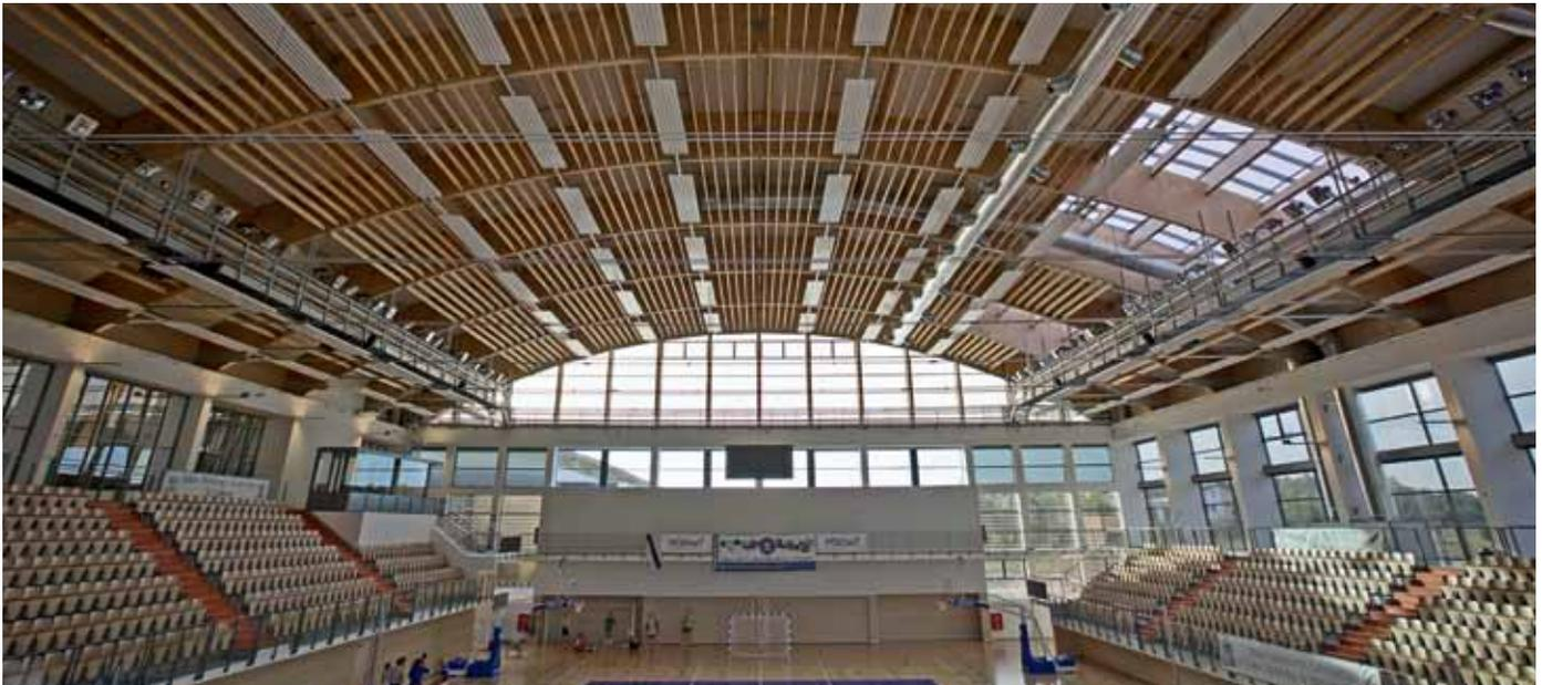
In order to heat the 5,000 m<sup>2</sup> large hall evenly and efficiently, the decision was made to choose Zehnder radiant ceiling panels. A total of 372 m<sup>2</sup> of perforated radiant panels for noise reduction were installed on the wooden structure which supports the roof of the hall.
