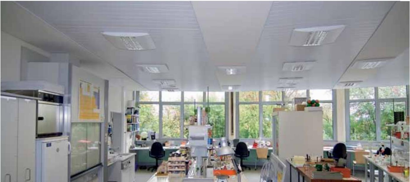
And the result was a lesson to all: the system was also installed in the chemistry area, in combination with a ventilation system. Inlets and outlets were integrated flush in the ceiling sails; the lighting was fitted on the sails.
