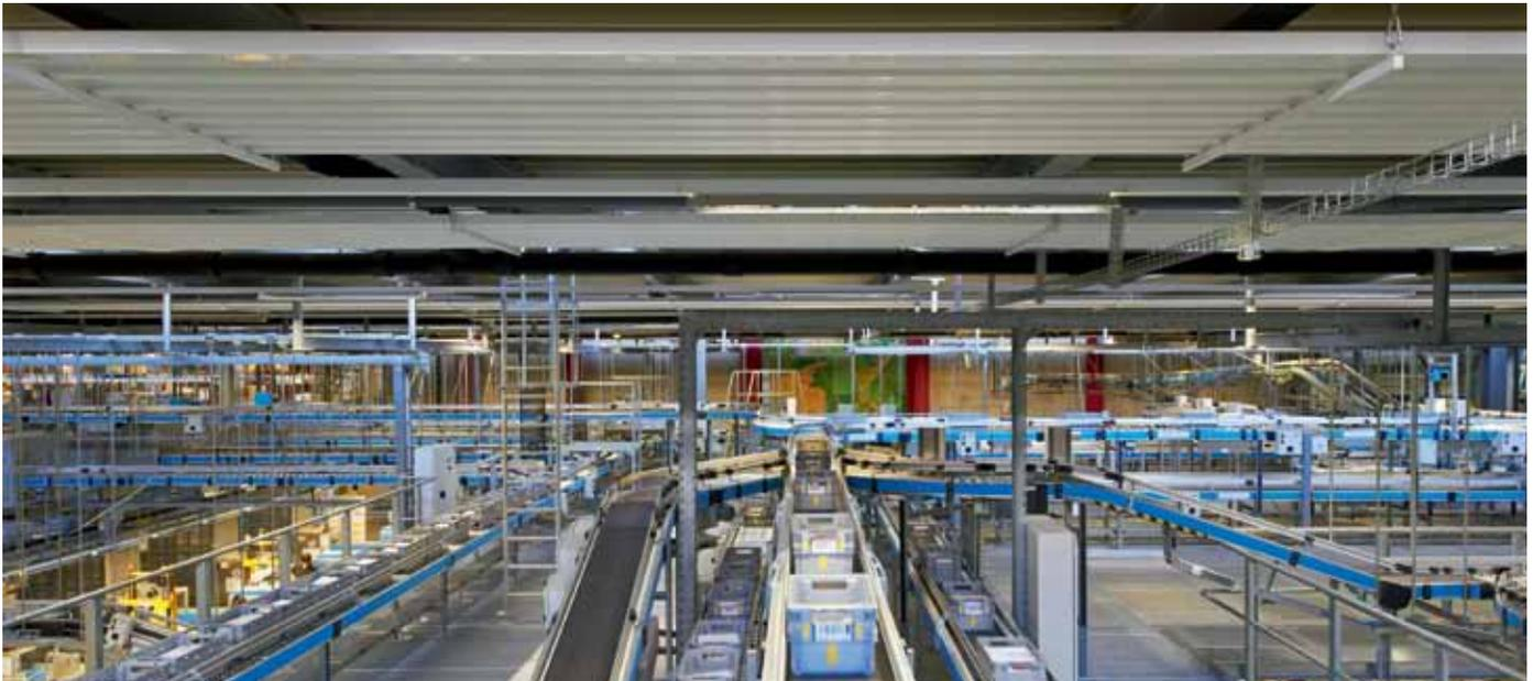
It is only logical that emphasis is also placed on having a high-performance system in the area of climate-control technology: With Zehnder radiant ceiling panels, the planners of the modern logistics center opted for pure efficiency.
