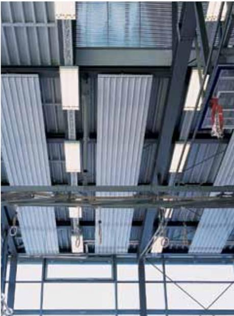
Twelve radiant ceiling panels from Zehnder were integrated flush with the ceiling along the entire length of the hall, fitted with precision down to the centimeter. Superimposed headers have also proven themselves since being installed, earning full marks for efficiency.
