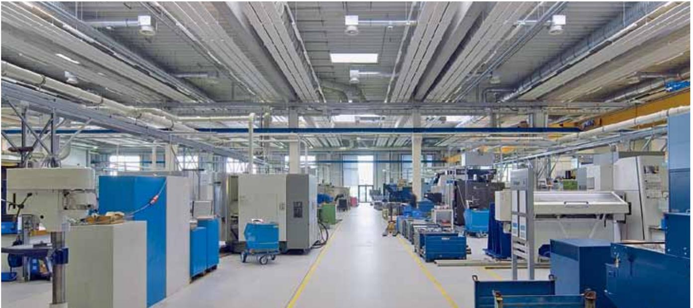
A combination of Zehnder radiant ceiling panel designs were utilized based on the individual department and its particular requirements. Ventilation outlets and lighting elements were integrated into the enclosed ceiling sails.
