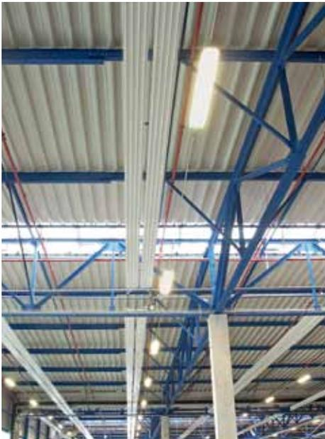
Emphasis is also placed on performance and efficiency in the area of climate-control technology, in the form of a Zehnder radiant ceiling system. 19 km of Zehnder radiant panels were installed.
