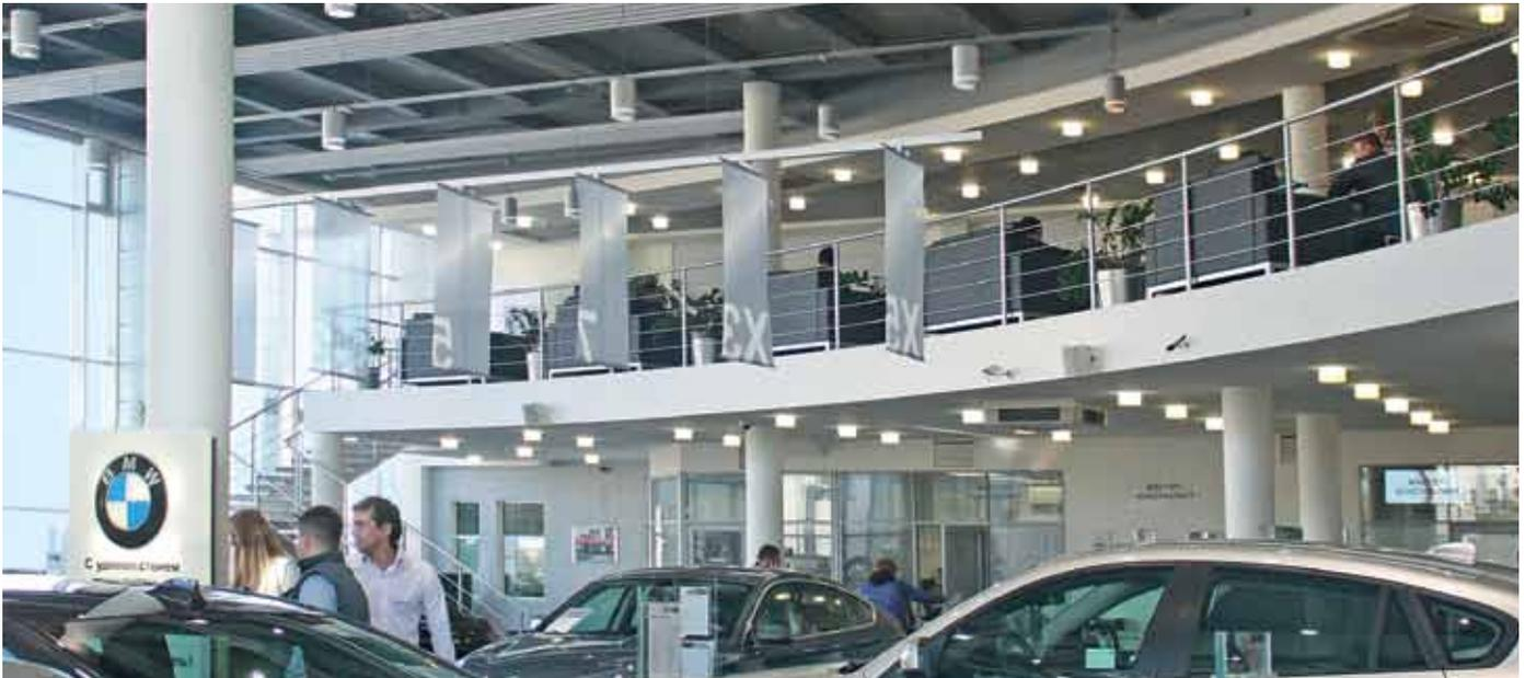
The Zehnder radiant ceiling system was selected in order to enable the best possible indoor climate conditions to be achieved in both the showroom and the workshop. A total of 150 m<sup>2</sup> of individual modules were installed.
