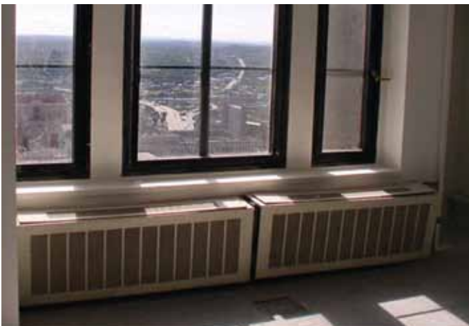
Before: Original induction units
