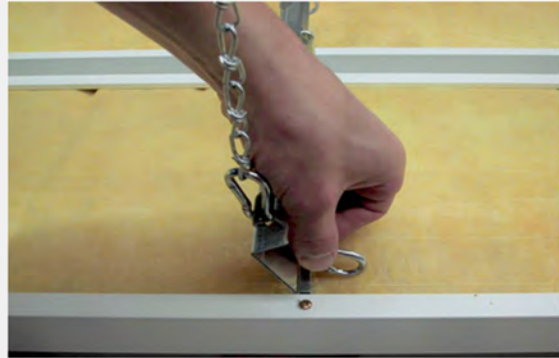
6. Connect the snap hooks of the multiple suspension bar to the installation hole of the mounting axis of the ZIP panel.
