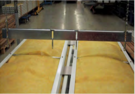
5. Mounting of chain and multiple suspension bar at the ceiling.
